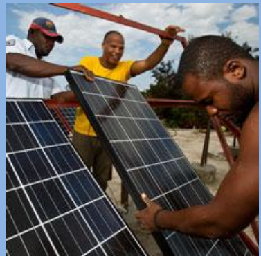
Top: Rotarian Florence Marc-Charles (right) and a volunteer doctor treat a 12-year-old patient with facial wounds during the medical mission. Bottom: Rotarian Christopher Castor (middle) and Haitian volunteers install solar panels to run a medical clinic and water well for a village on the island of La Gonave, Haiti. Rotary Images/Alyce Henson
